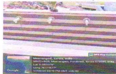
Push tap for reduce water consumption
